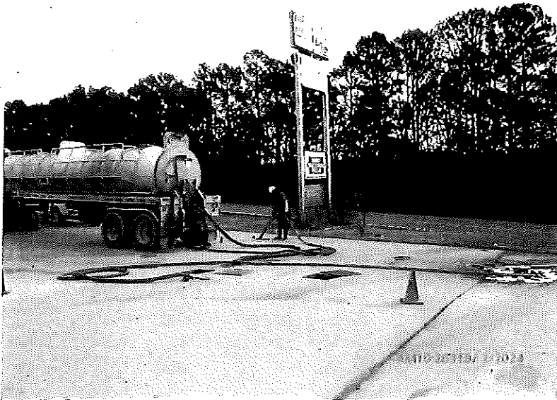
Close up of fuel/water evacuation process on February 2, 2024.
